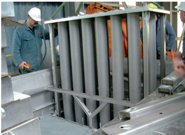
Installation of filter elements.
